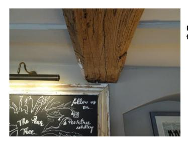
Photo 2. A downstand beam found on the ground floor
