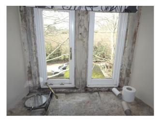
Photo 3. Stone mullioned window with ovolo mouldings found on the attic floor
